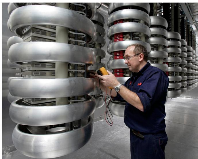
Maintenance being undertaken on state of the art power electronics which is housed in a HVDC Converter Station.
